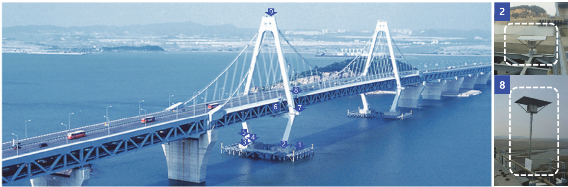
Fig. 1 The locations and photos of salinity measurement devices in the Youngjong Bridge
