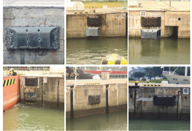
Fig. 10 Synthesis of fender images with barnacles and engraving lines
