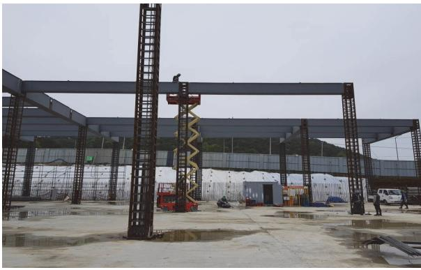
**Fig. 1** Construction of frames using NRC structural system
