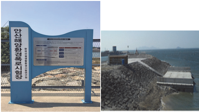
Fig. 2 The view of marine environment exposure test site
