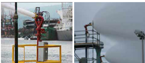
Fig. 1 Installation of fire fighting monitor
