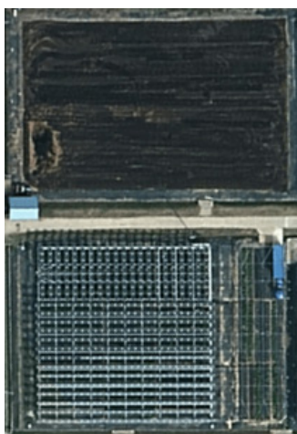
<Figure 6> An Satellite Image of the Subject APV System in Naju-si, Jeollanam-do, South Korea
