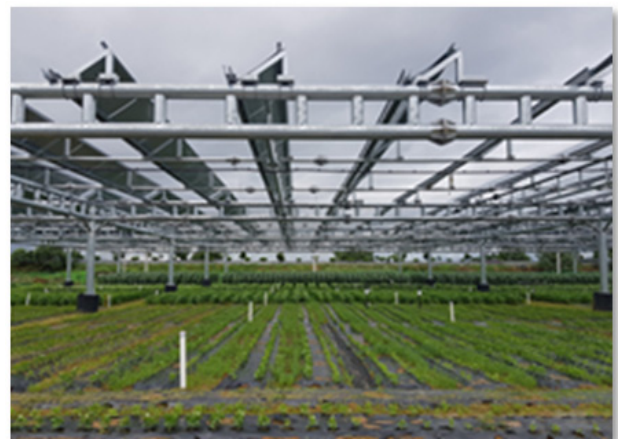
<Figure 1> Agrophotovoltaic System [10]
