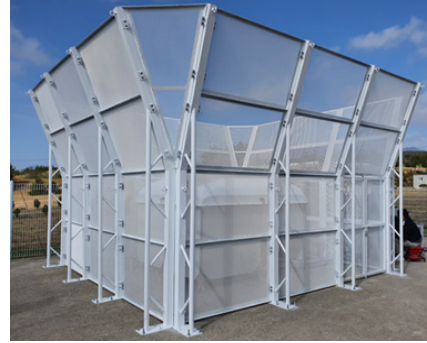
<Fig. 12> Manufactured Clutter Fence
