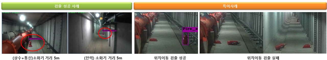
Fig. 5. Application of fire extinguisher object detection model in underground utility tunnel
