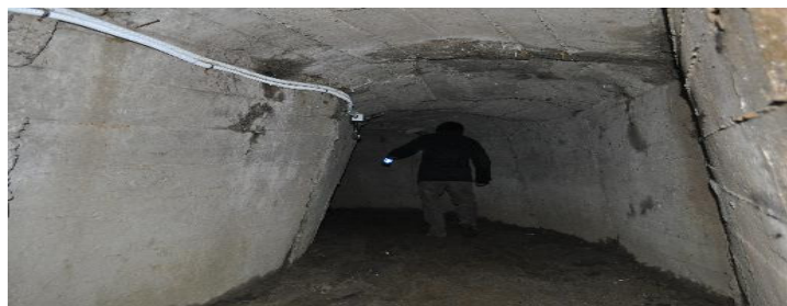
Fig. 6. Additional lining installation inside small-scale tunnels
