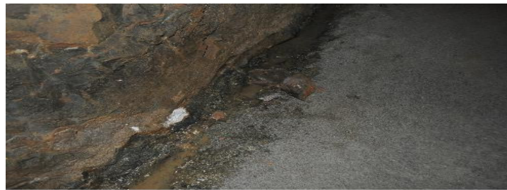
Fig. 8. Discharge of ground water inside small-scale tunnels
