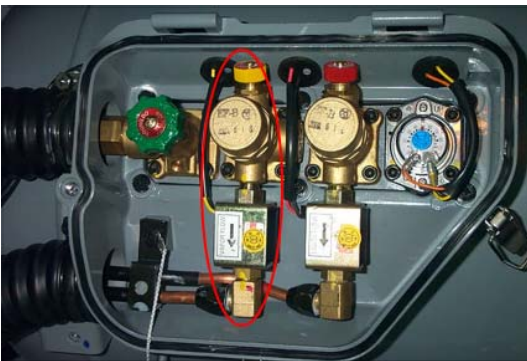
Fig. 5. Emergency cutting gas solenoid valve of LPG a car
