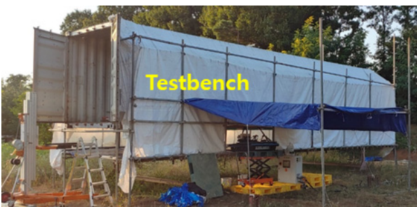
Fig. 12 Testbench using a container
