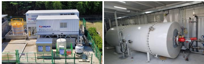
(a) Bird-eye view of SF 6 decomposition and control system (b) Incinerator for SF 6 decomposition
