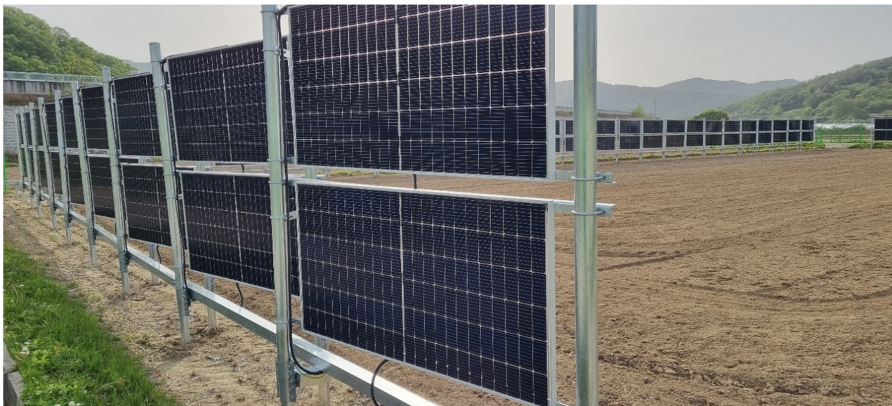
Fig. 3. Application of Fence type bifacial PV system installed at Kyungpook National University's agricultural field in Korea
