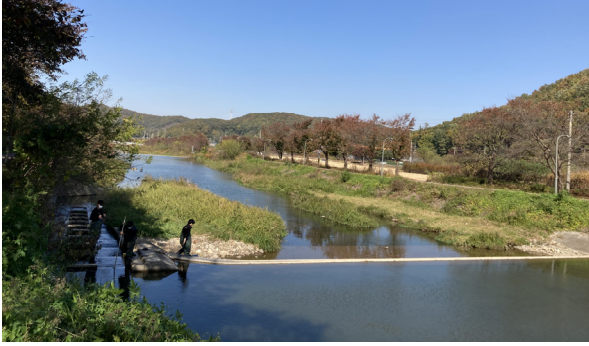
(b) Fishway located at left bank
