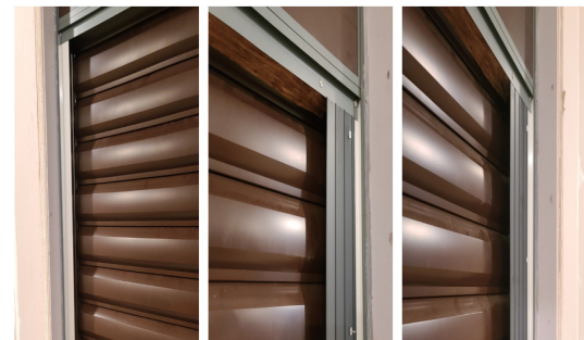
Fig. 6. (Color available online) Bracket width installation.
