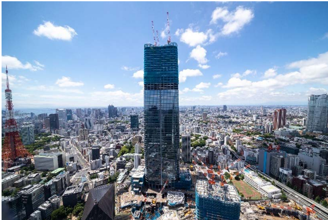
Figure 21. The current construction situation.
