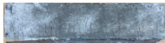
Fig. 12 Cracking picture of specimen strengthened with carbon fiber sheet
