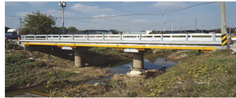
(b) After reinforcement
