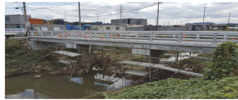
(a) Before reinforcement
