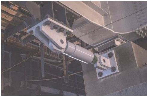
Fig. 4 Shock absorber
