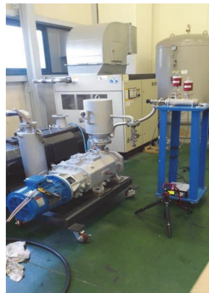
(b) The measuring equipment setting
