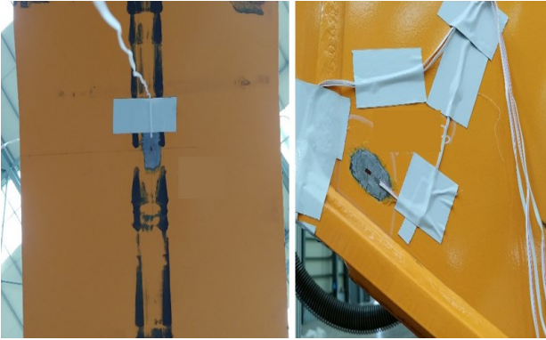
Fig. 1 Example of strain guage measurement for structural damage
