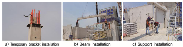
Fig. 4. Construction procedure for beam installation
