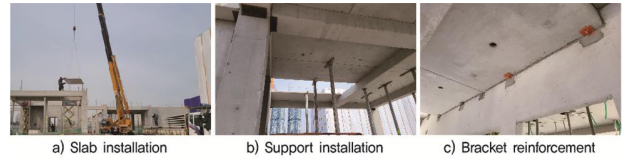
Fig. 6. Construction procedure for slab installation
