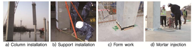
Fig. 3. Construction procedure for column installation
