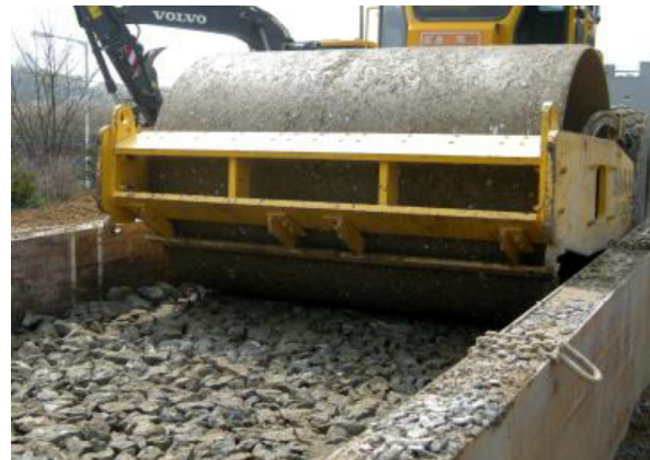
(b) Compaction for test
