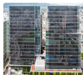
Fig. 3. BIPV Installation Case of Euljiro Twin Tower in Seoul
