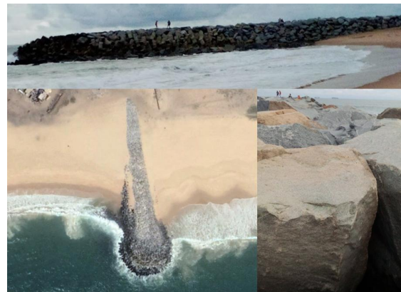
Fig. 14. One of seven groynes built in 2013 as a technical measure.
