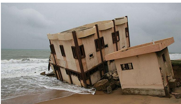
Fig. 11. Damaged hotel infrastructures by coastal erosion (Ocean Climate Alliance).
