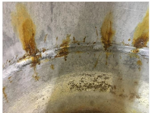
Fig. 2. Example image with visible corrosion, stress corrosion cracks, and artifacts (scratches, shadows, etc.). Note: this is a laboratory corroded stainless steel sample and not an image from an actual used fuel canister; to the best of our knowledge no canisters have been detected with defects).
