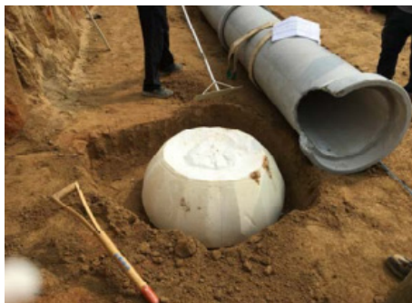
Fig. 5. Pipe and cavity for test
