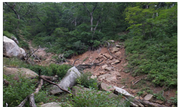
Fig. 2. Slope failure of granite weathered soil (Seoraksan Mt.)
