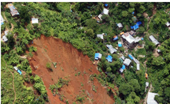
Fig. 1. Slope failure of gneiss weathered soil (Jirisan Mt.)
