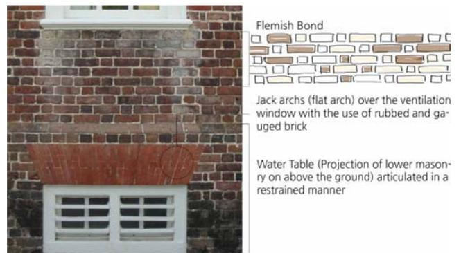
Fig. 7. Detailing of the manner of brickwork in the Wythe's House
