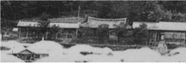
Fig. 8. Building presumed to be Gaegsa (1950)
