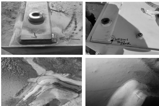
Fig. 17 Real failure cases
