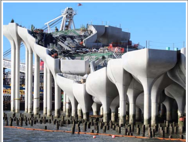
b: Heatherwick studio pier 55 hard landscape construction
