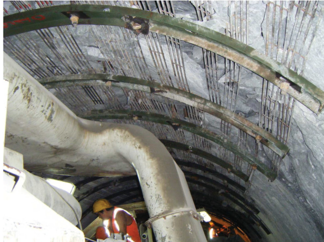
Fig. 3. McNally TBM support system (Brox, 2013)
