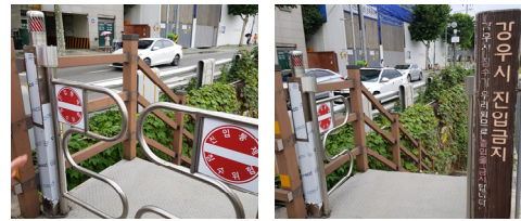
Fig. 11. River entrance blocking facility
