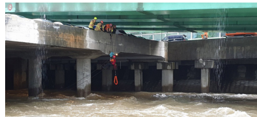
Fig. 12. Gurogyo at the time of flood accident (2019.9.5., by Gwanak fire station)
