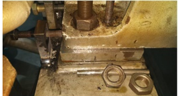
Fig. 15 Adjustment of inter. bearing height with shim plate
