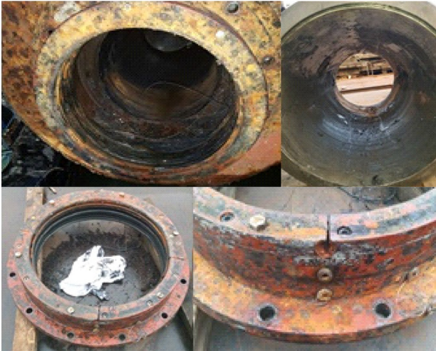
Fig. 3 Aft stern tube bearing and seal box damage
