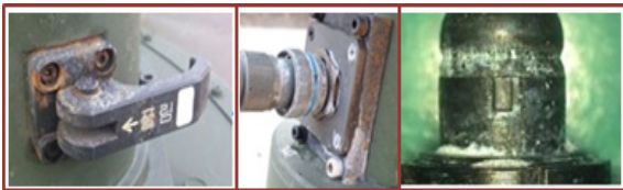
Fig. 1. Corrosion of mechanical structure
