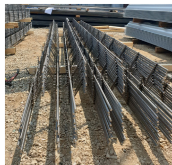
(b) Carry-in pre-fabricated rebar
