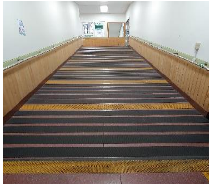
Figure 3. Ramp of the target building
