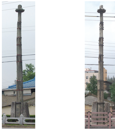
(a) Before Restoration (b) After Restoration
