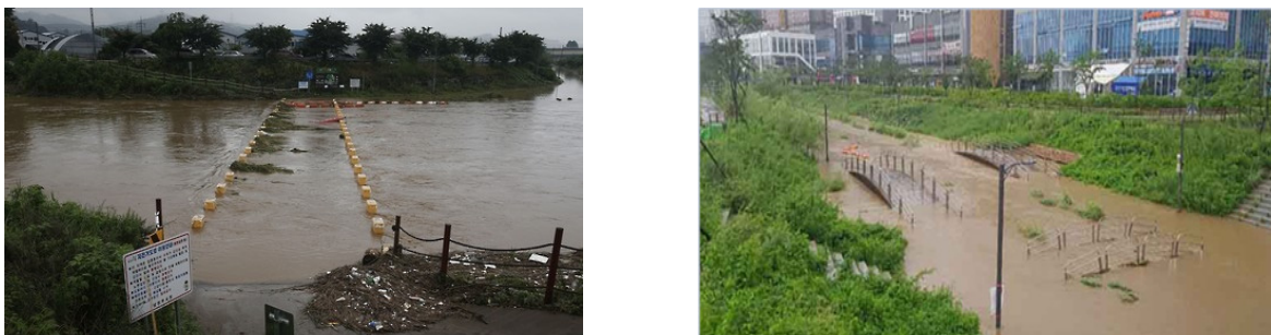
Fig. 1. Rivers with poor maintenance during flood season (Left: Wangsuk river, Right: Mangwal River)
