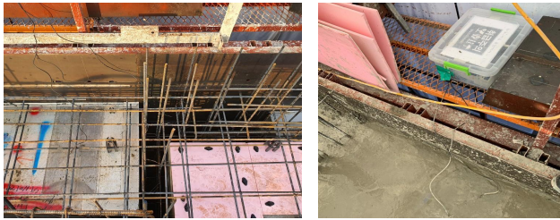
Figure 6. Installation of CIMS
