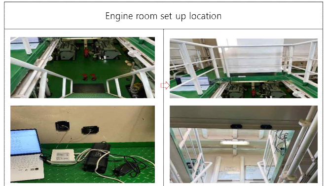
Fig. 13 Change the setup location in the Engine room
