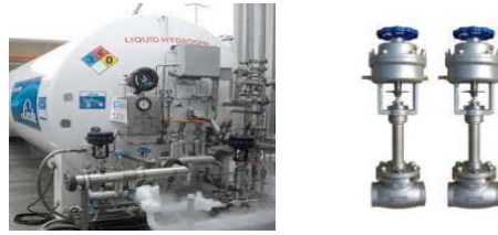
Fig. 4. Example of Liquefied Hydrogen Emergency Shutoff Valve.
