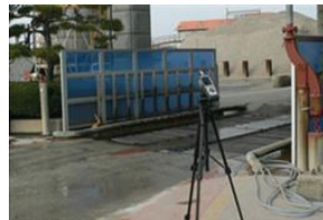
(b) Wheel-washing facility
