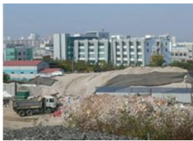
(b) Aggregate yard(north)
