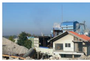
(c) Industrial facilities(west)
