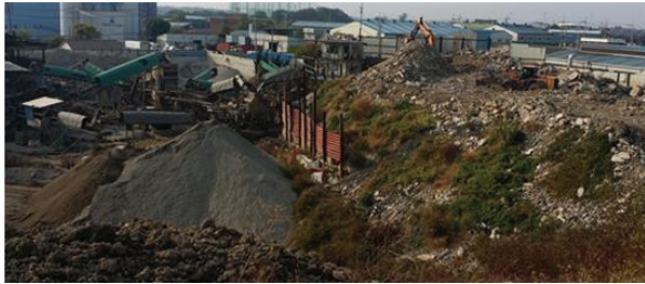
(a) Waste treatment facility(northwestward)
