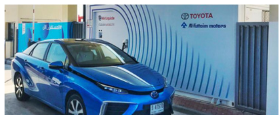
Fig. 2. First hydrogen station in UAE 2)
