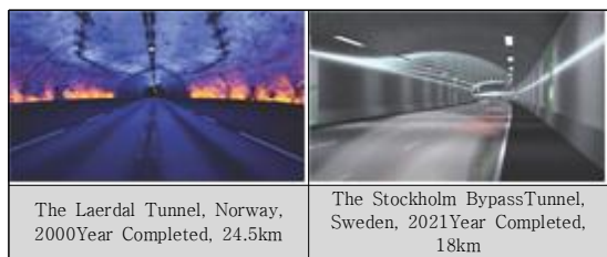
Fig. 1. Lighting installation status in overseas tunnels
