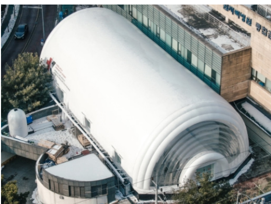
(b) Air-beam pavilion (Seoul, 2021) : Double-layered pneumatic membrane ( http://bare.kr/archive/29 )
