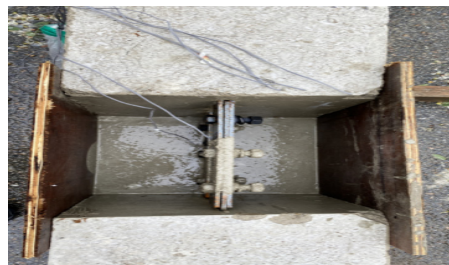
(b) Injection of non-shrink mortar
