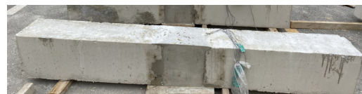
(c) Removal of concrete form
