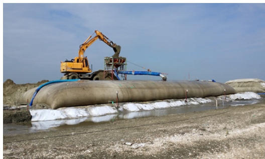
Fig. 1. Geotextile tube filled on land
