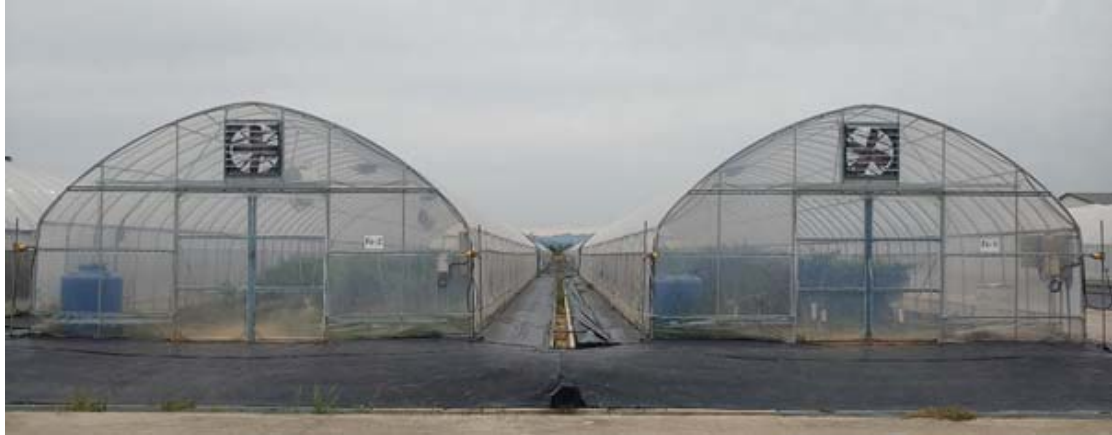
Fig. 1. Plastic green houses that control temperature using a ventilation system. (M) maintained at more than 15°C (L) treated with low temperature using ventilation system from May 2 to May 27.
