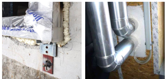
(a) Window and Wall Junction (b) Pipes on the Wall
